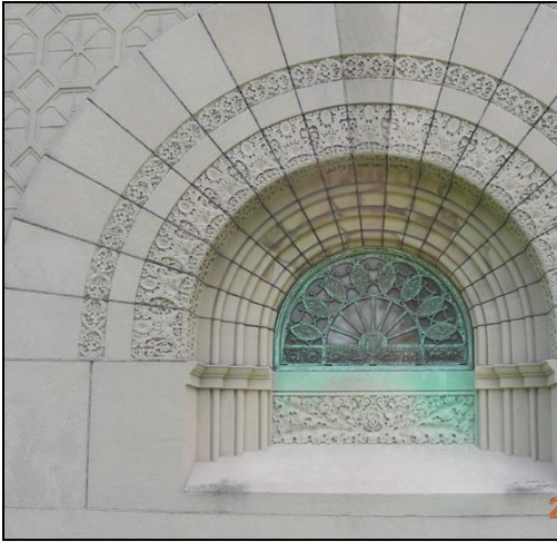
Figure 5. Intricate sculptural detail in the Indiana Limestone of Louis Sullivan's Getty Tomb in Graceland Cemetery, in Chicago's Lincoln Park district. Note the staining of the central stone panels from the weathering of the bronze window grille above it. This is a deposit of copper (II) carbonate hydroxide caused by the bronze reacting to atmospheric water and carbon dioxide. The classic malachite greenish-blue is usually considered an ornamental asset of weathering bronze, but in this case, it has adversely affected the stone beneath it. (Photo by author)
