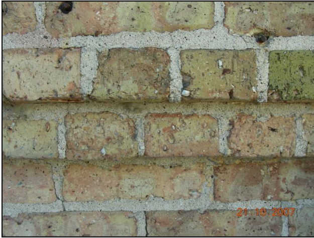
Figure 1. Detail of glacial-till-derived, nineteenth-century brick in Geneva’s old city power plant. Note the pebbles of dolostone and chert embedded in the fired clay. While most Chicagoland brick is made from lakebed deposits of uniformly small particle size, this coarse, fruitcake texture and more variable color range provide more visual interest. Each brick has its own geologic story to tell and is not just an anonymous building block. (Photo by author)
