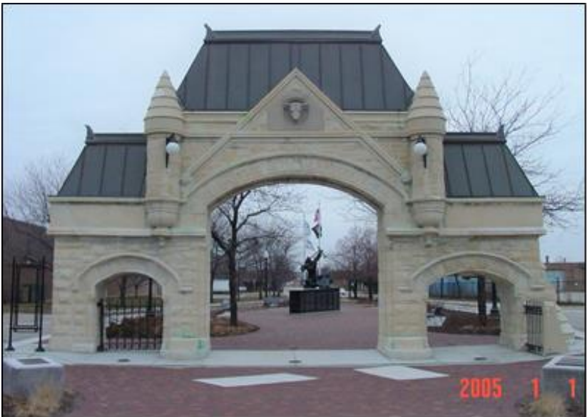
Figure 4. Chicago's Union Stockyard Gate, an excellent example of the ornamental use of Chicagoland's local Silurian dolostone. This 420 Myo sedimentary rock, still a very common sight throughout the region's built environment, was mostly quarried in Lemont and Joliet. It hit its peak of popularity with architects before the mid-1890s. (Photo by author)
